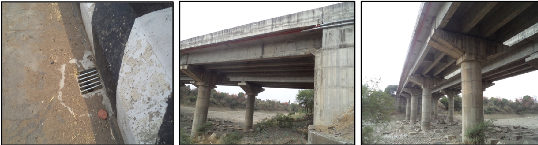
Fig 3.109B: MjB at Ch. 77+850 -Drainage spout, View of underside of superstructure of bridge
