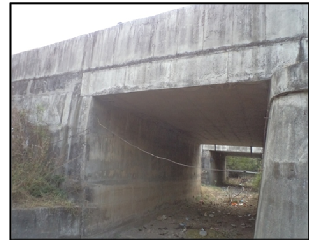
Fig 3.127: MnB at 140+205 – View of deck slab, minor vegetation in quadrants, view of underside of bridge
