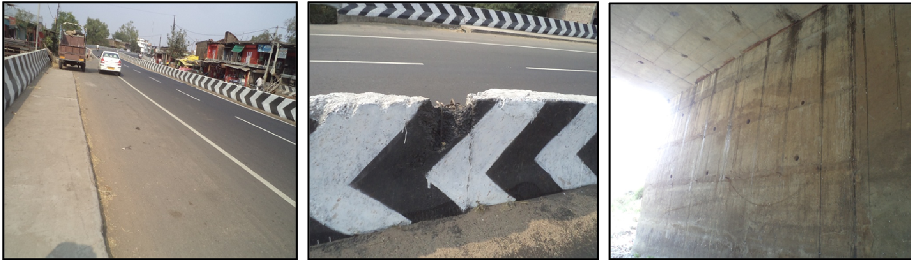
Fig 3.118: MnB at 67+420–View of deck slab, minor damages in crash barrier, underside of box
