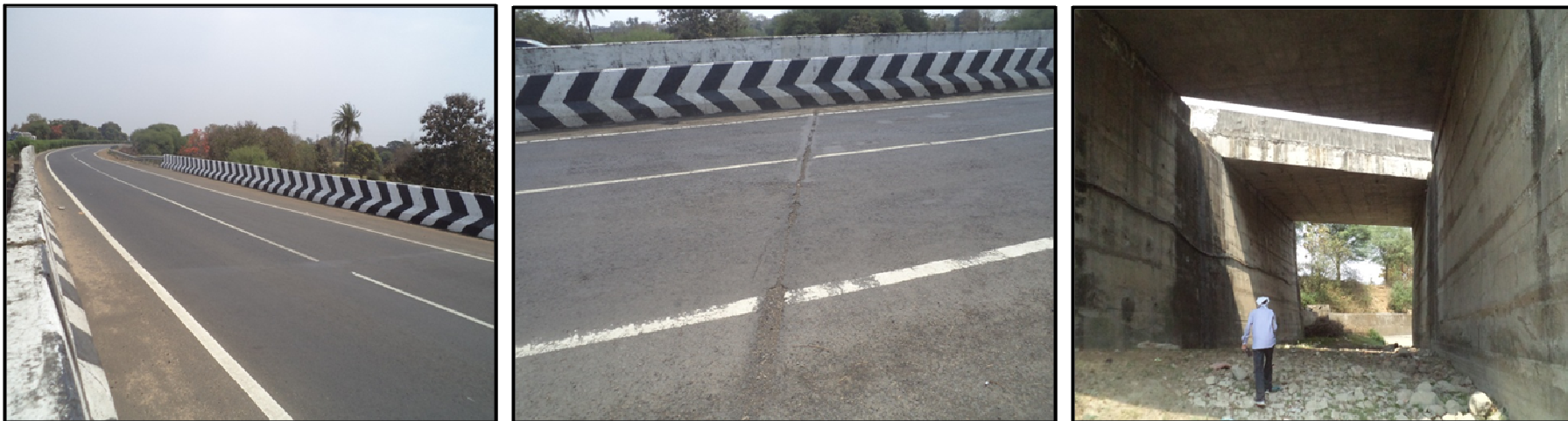
Fig 3.121: MnB at 105+190-View of deck slab, Minor repairs required on expansion joints, view of underside of bridge
