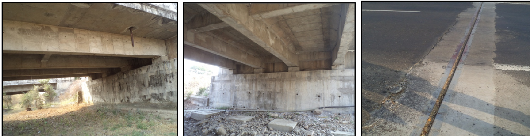
Fig 3.116: MnB Ch.60+970–View of underside of bridge, condition of expansion joints
