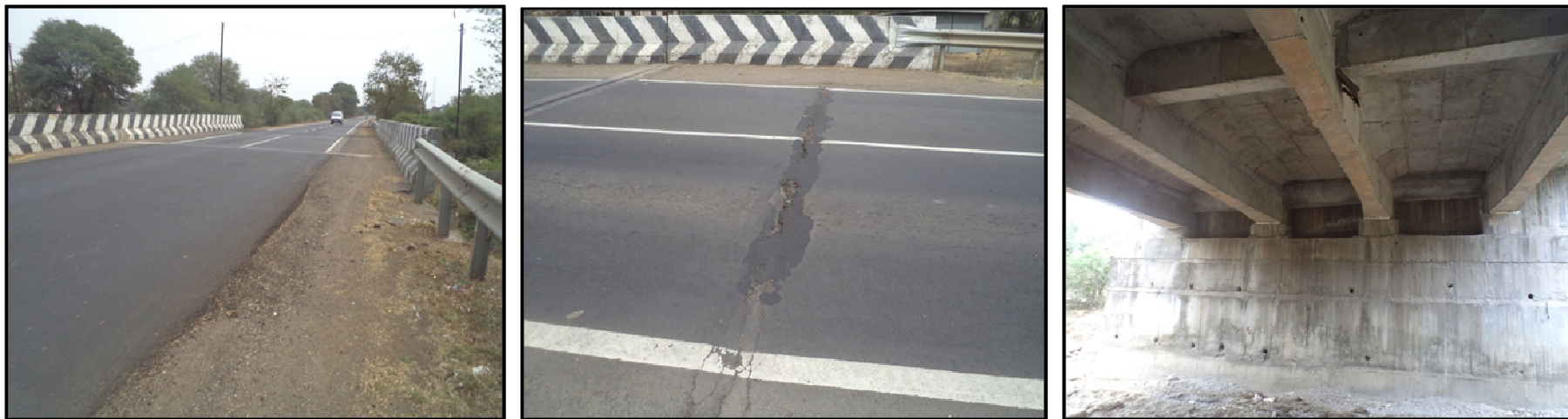
Fig 3.123: MnB at 117+960 - Condition of approaches, expansion joints buried, view of underside of bridge
