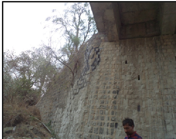
Fig 3.111B: MjB at Ch 128+510–Vegetation on abutments, minor repairs of substructure underway
