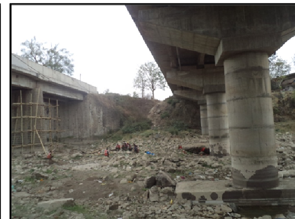
Fig 3.111B: MjB at Ch 128+510–Vegetation on abutments, minor repairs of substructure underway
