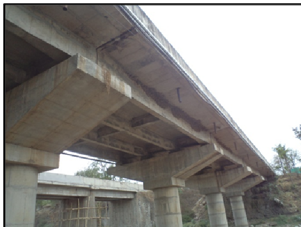
Fig 3.111B: MjB at Ch 128+510–Vegetation on abutments, minor repairs of substructure underway
