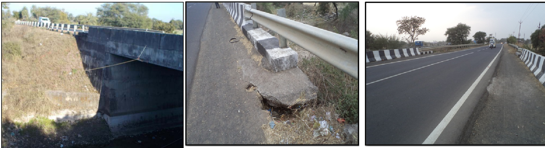
Fig 3.115: MnB Ch.45+250–Status of quadrant pitching & toe wall, erosion of embankment, view of deck slab
