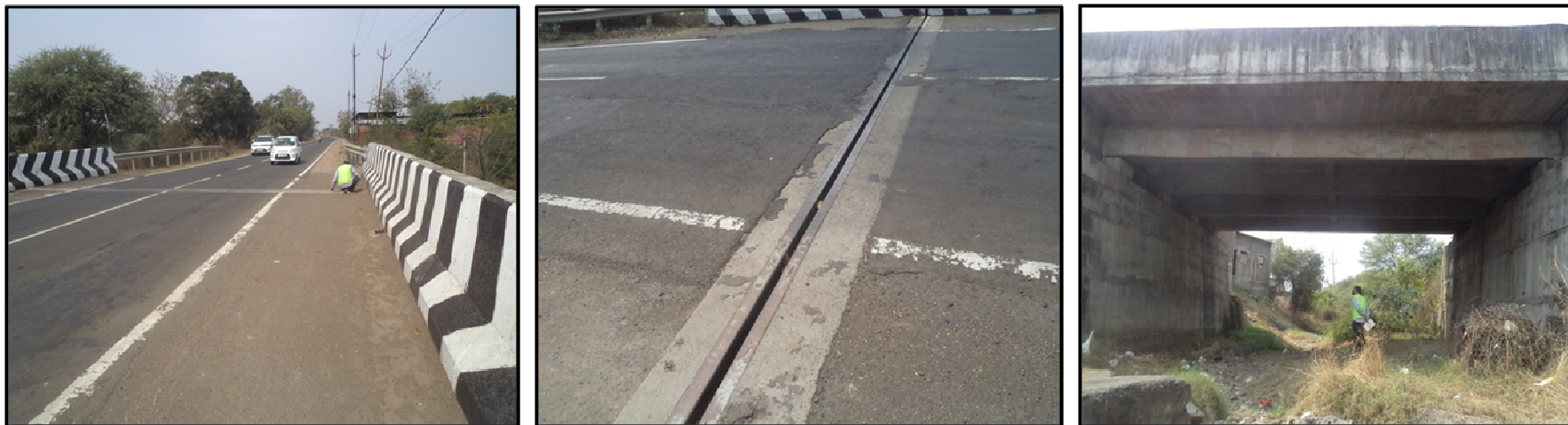
Fig 3.124: MnB at 122+860–View of deck slab, condition of expansion joint, view of underside of bridge
