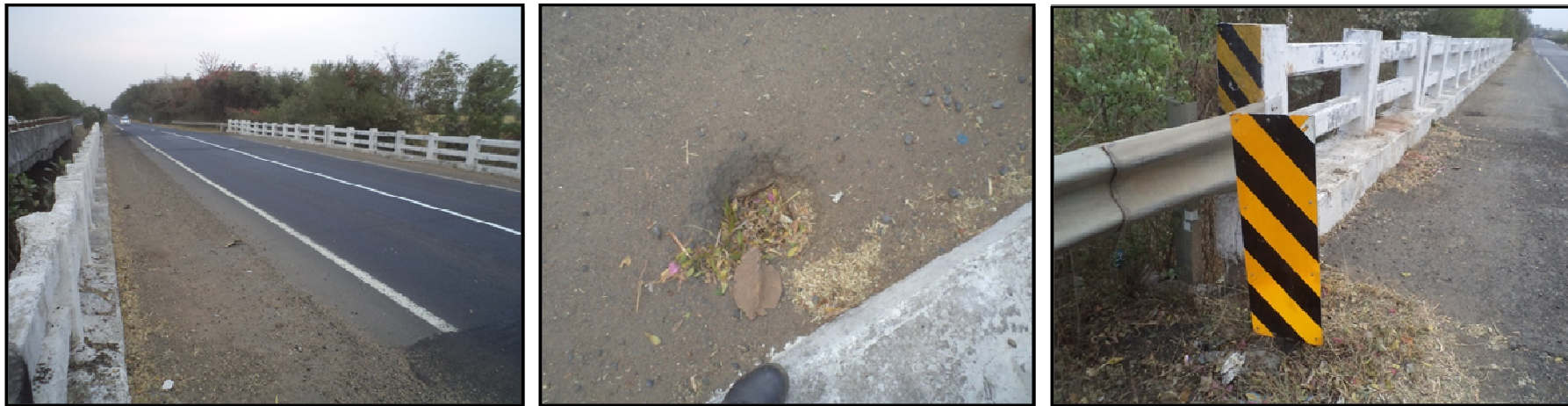
Fig 3.114: MnB Ch.38+850–View of deck slab, drainage spout cleaning required, hazard marker
