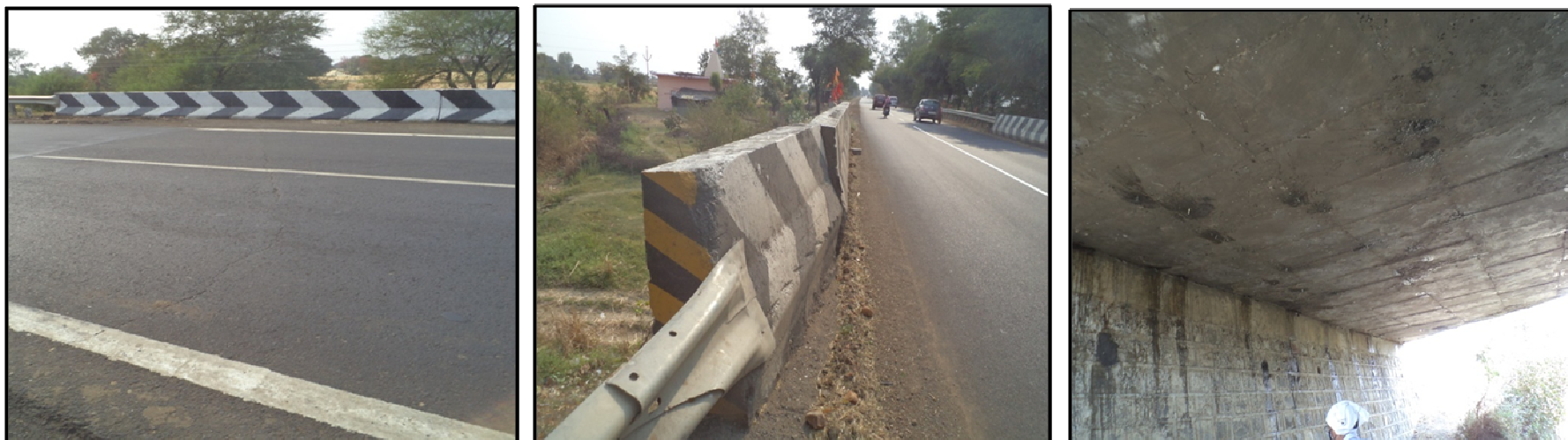
Fig 3.117: MnB Ch.63+550 – View of deck slab, minor damages in crash barrier, view of underside of slab
