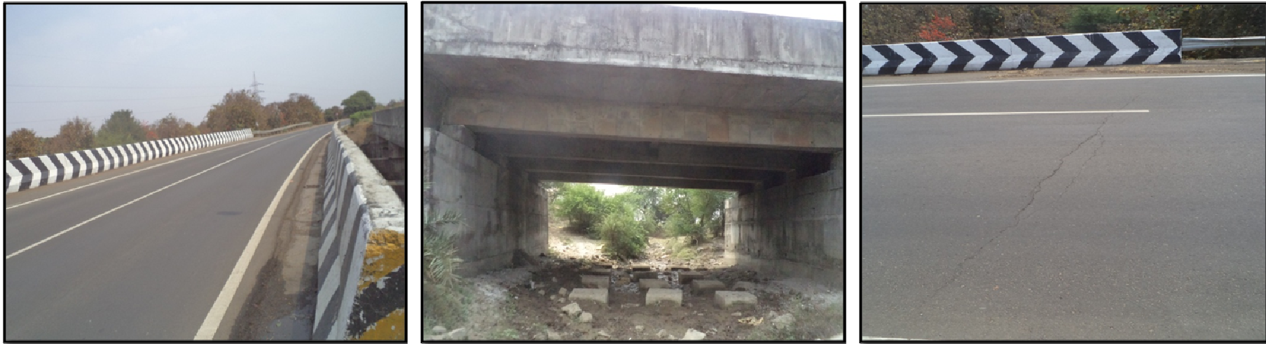
Fig 3.122: MnB at 107+900-View of deck slab and underside of bridge, expansion joints buried
