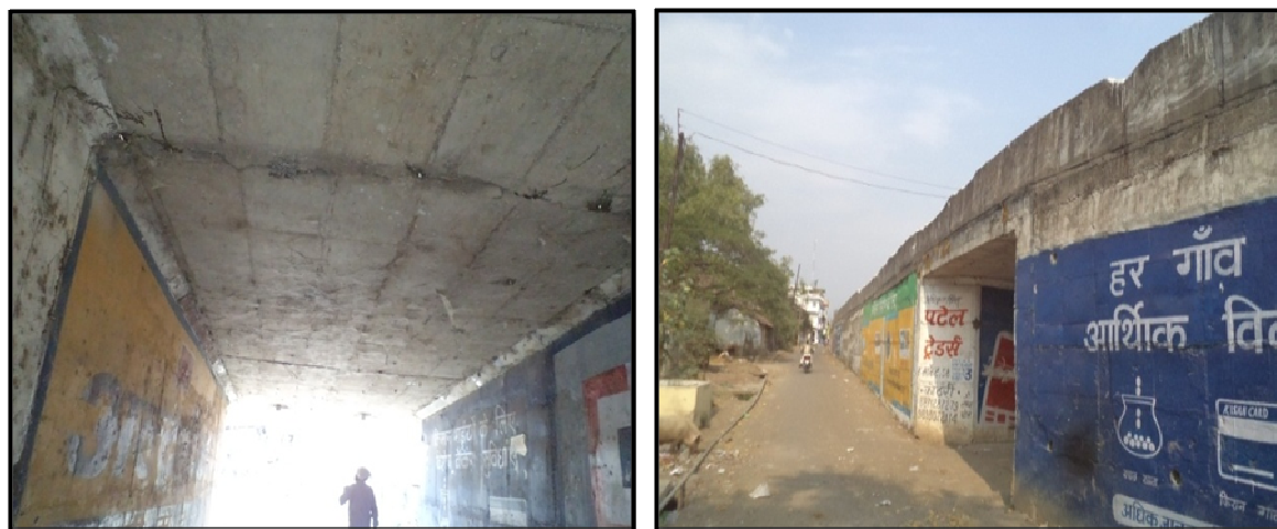
Fig 3.130: PUP at 67+250–View of underside of PUP, minor damages in crash barrier
