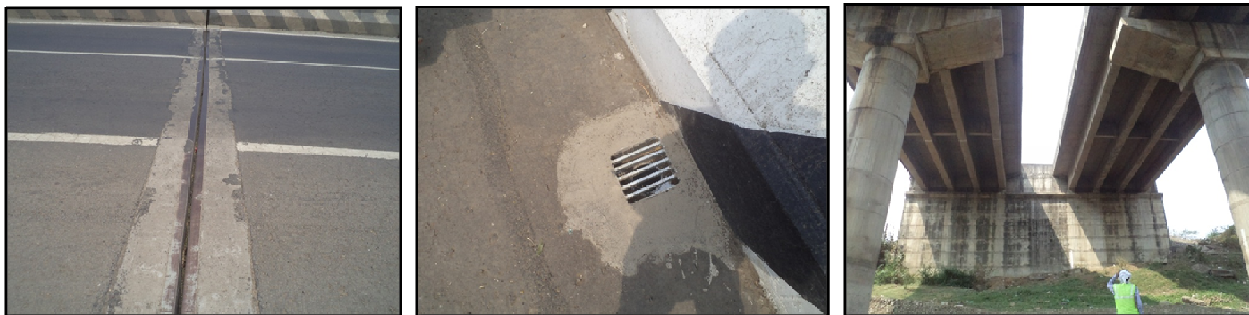
Fig 3.110B: MjB at Ch 121+120–Expansion joints & drainage spout, underside of superstructure of bridge
