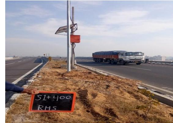
Fig 4.230: Camera with solar panel at Ch 51+400
