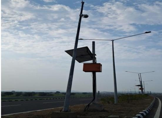
Fig 4.234: Camera with solar panel at Ch 2+250
