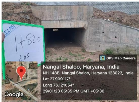
Fig 4.385: Box Culvert at Ch 1+800 LHS
