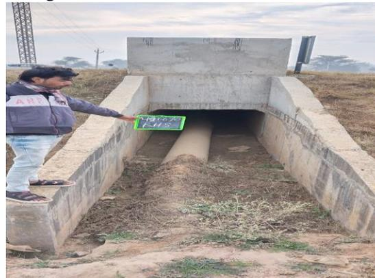
Fig 4.368: Box Culvert at Ch 49+670 RHS
