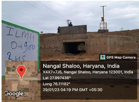
Fig 4.382: Box Culvert at Ch 0+900 RHS
