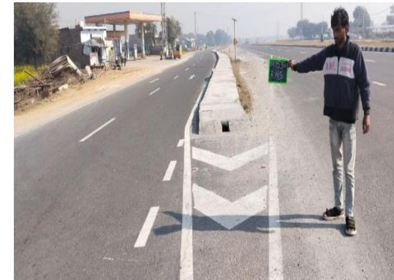
Fig 4.183: RCC Toe Drain at Ch 52+550 RHS
