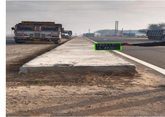
Fig 4.180: RCC Drain at Ch 48+130 LHS
