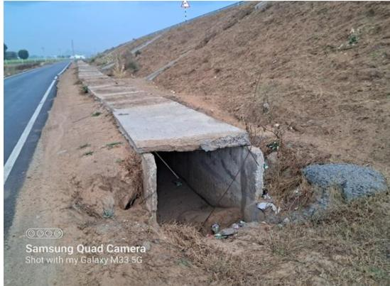
Fig 4.190: RCC Toe Drain at Ch 1+600 RHS
