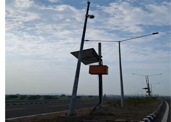
Fig 4.236: Camera with solar panel at Ch 2+250
