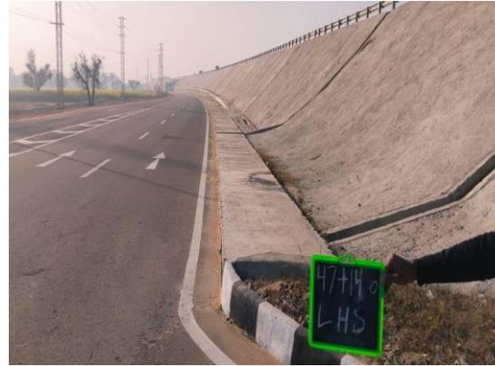
Fig 4.179: RCC Toe Drain at Ch 47+140 LHS
