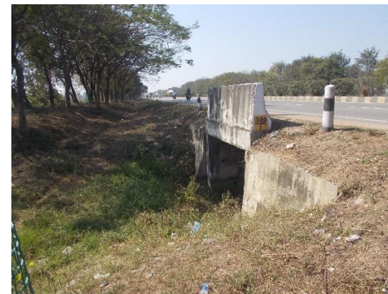
Fig. 4.105 : Box Culvert at Ch. 308+214
