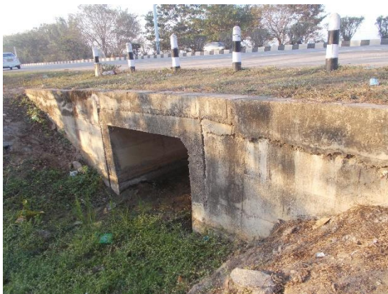
Fig. 4.100 : Box Culvert at Ch. 286+917
