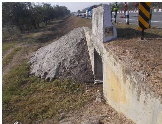
Fig.4.104: Slab Culvert at 301+387
